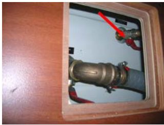
House water inlet: Plumbing board
