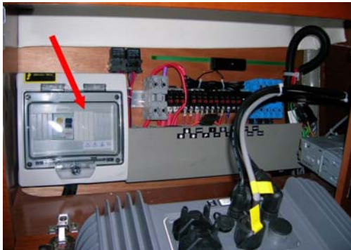
Differential switch 40A - Chart table unit
