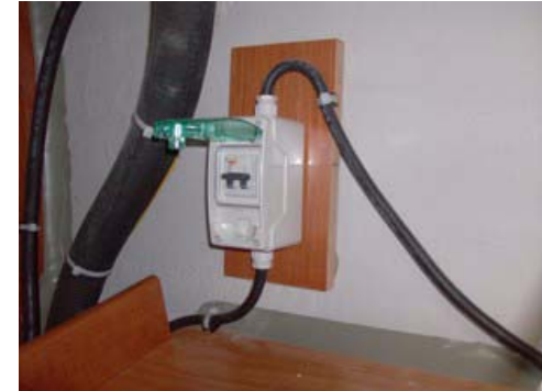
Bipolar circuit breaker 32A Cockpit locker - Starboard (Ref 2)
