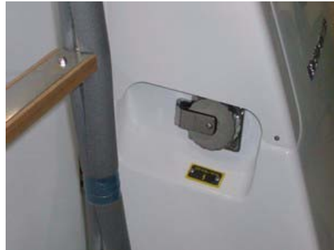
Shore power socket 220V - 30A (Ref 1)
