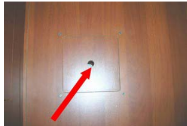
House water inlet: Plumbing board
