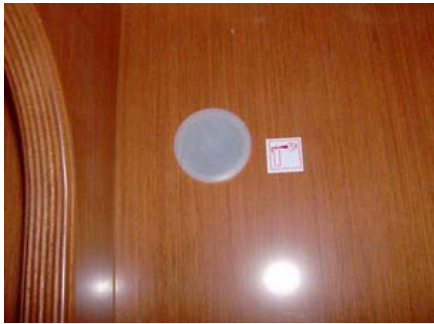
Extinguisher hole located under the companionway step
