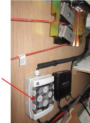
Ref 2: Bipolar circuit breaker (Protection)
