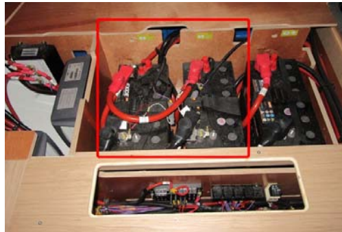
Service batteries: 2 x 120A
