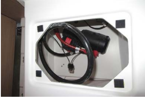
Access to the engine: Aft cabins
