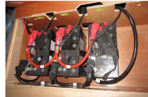
Spare service batteries: 3 x 100A
