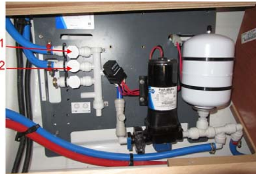
Water tank selection valves
