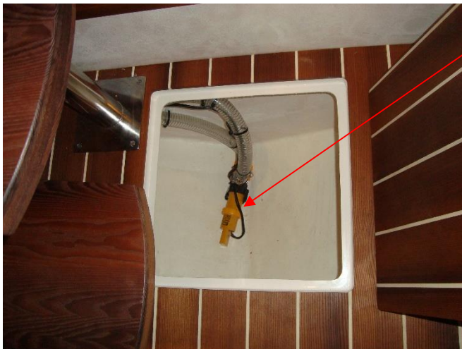
Front automatic bilge pump and front intake for manual bilge pump
