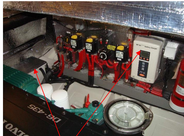
Start battery and charger located in engine room
