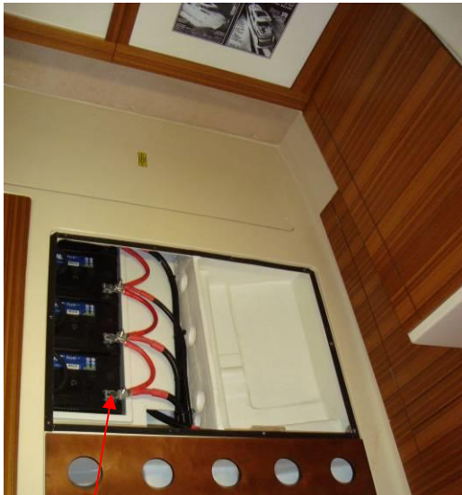
Service battery bank located in aft cabin under bed
