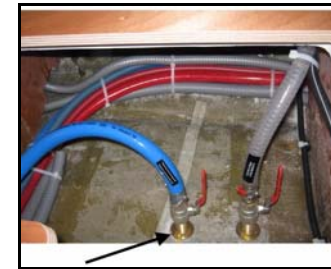
Seawater inlet (Reference 3)
