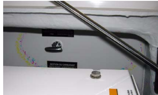
Lever pushed: Supply Diesel - Starboard tank
