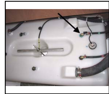
FUEL SUPPLY VALVE
