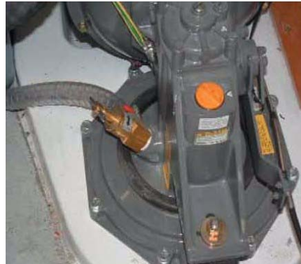
ENGINE WATER INTAKE VALVE VIEW INTERIOR
