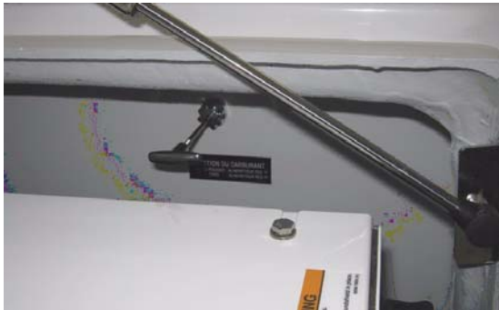
Lever pulled :Supply Diesel - Port tank
