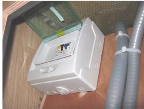
220V BREAKER Location: Port aft cabin
