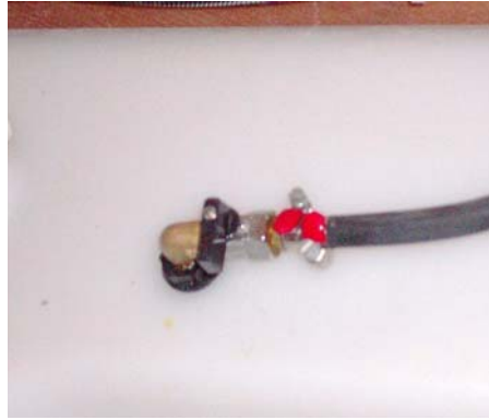
FUEL VALVE LOCATED ON THE FUEL TANKS
