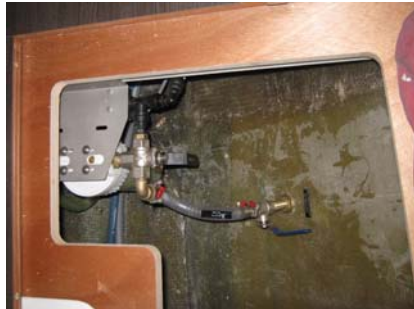
Seawater intake valve (Reference 2)
