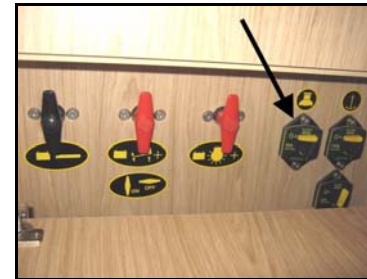
WINDLASS CIRCUIT BREAKER - 100A
