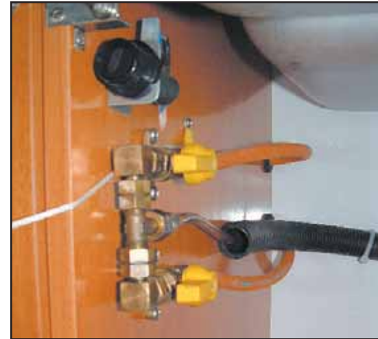
GAS VALVES (Locker to right of oven)
