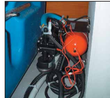
WATER PUMP + EXPANSION CHAMBER
