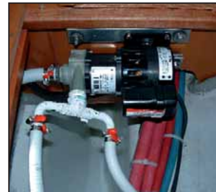
SEA WATER PUMP FOR AIR CONDITIONING
