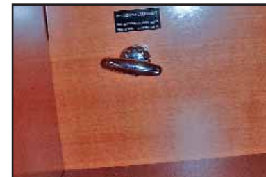
PULL-SWITCH FOR TRANSFER
