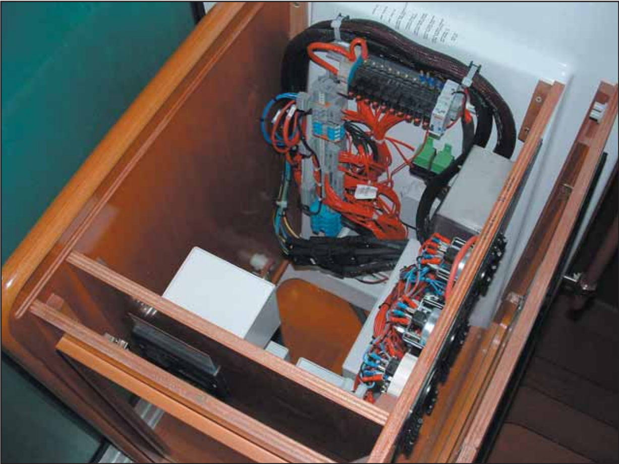
LOCATED BEHIND THE ELECTRICAL PANEL
