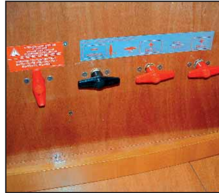
PORT AND STARBOARD AFT CABIN BATTERY SWITCHES
