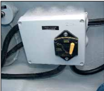
WINDLASS CIRCUIT BREAKER (FORWARD COCKPIT LOCKER)
