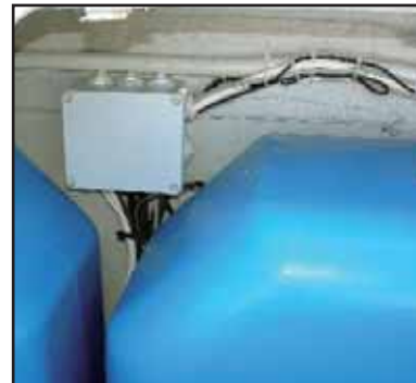
MAST JUNCTION BOX
