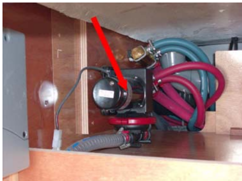
Aft electric bilge pump Location - Starboard cockpit locker Capacity: 15 litre / minute
