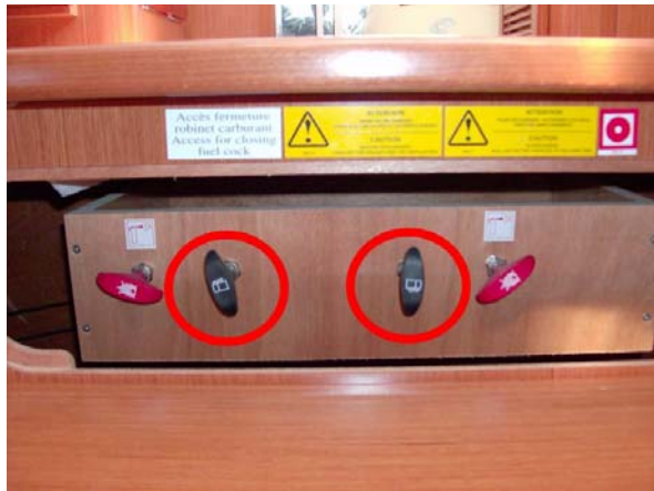
Remote valve shut off controls (Reference 2)
