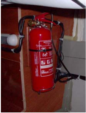
Fixed position extinguishers (Reference 1) - Engine compartment
