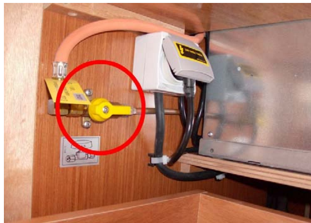
The valve is located under the kitchen cupboard
