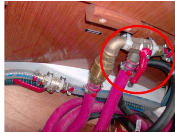
Selection valve - Shore fresh water / On board water circuit Location: Under the companionway
