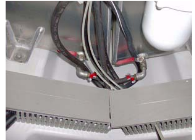
Tank interconnecting valve
