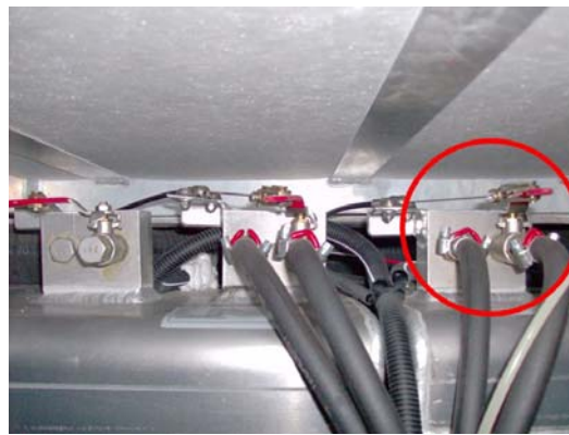
Engine supply valve on starboard tank (Reference 2)
