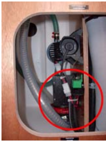
Forward electrical bilge pump Location - Under the companionway Capacity: 15 litre / minute
