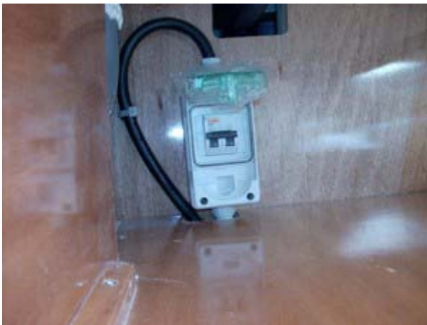
Breaker 30A 220V Cockpit locker Port side
