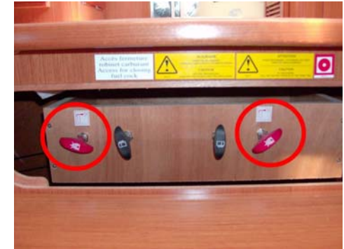
Extinguisher remote pull-switch (Reference 2)
