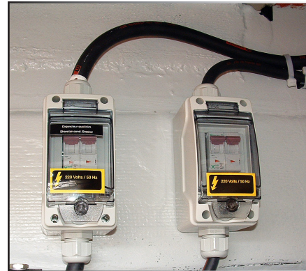
AUTOMATIC BREAKERS OF THE SHORE POWER SOCKETS
