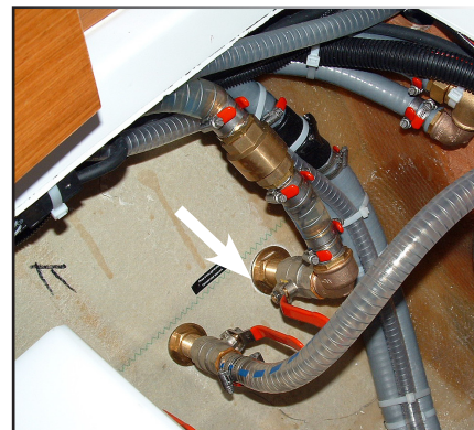
WATER INLET VALVE OF THE GENERATOR
