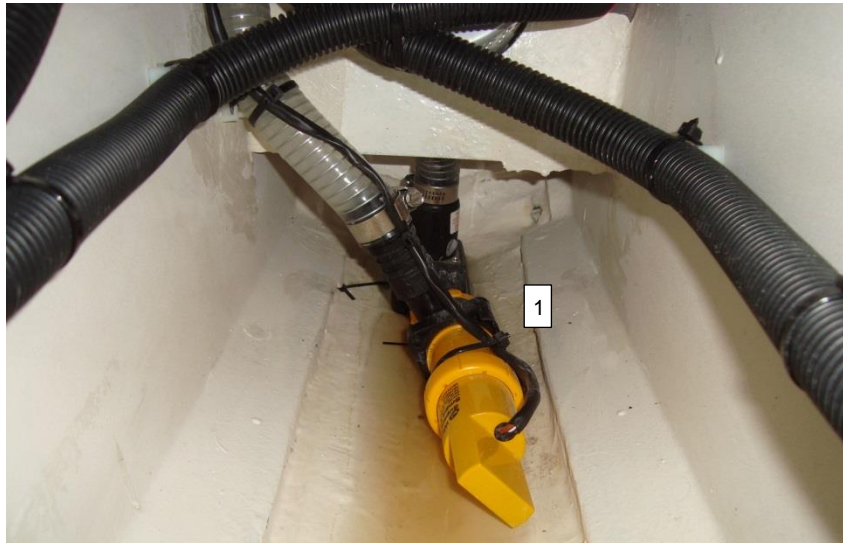
Picture 18: The automatic lensing system in the engine room (1)
