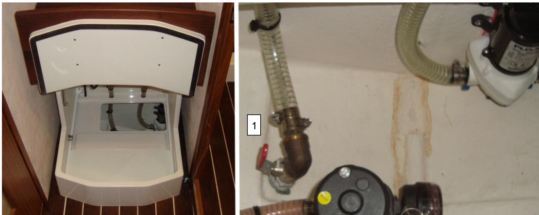
Picture 10: Location of the seawater inlet for toilet flushing (1)
