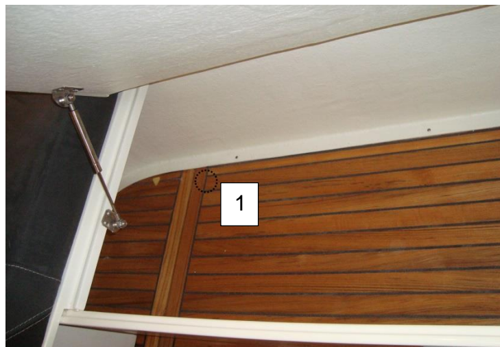
Picture 16: Aft deck drain on the port side (1)
