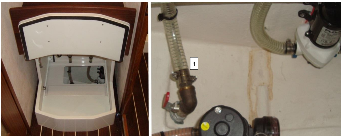
Picture 49: Bottom valve "open" (1).
